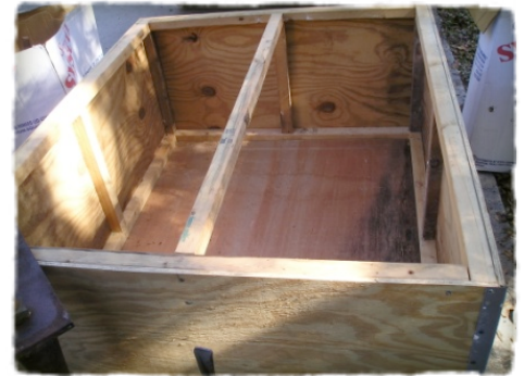
The crate is built...
